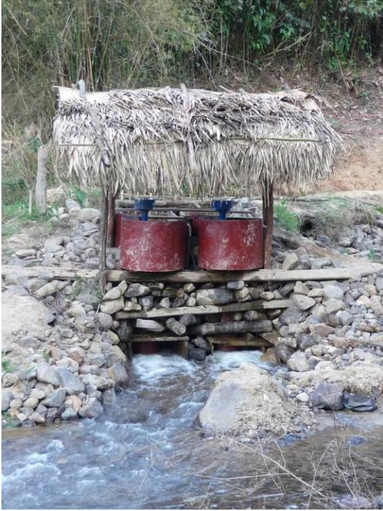
**Two 1 kW pico-hydro turbine units are installed to supply 24-hour electricity to 24 households plus communal buildings**
