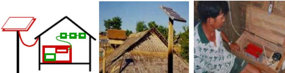
**Figure 3-3 Rent-to-buy solar home systems consist of solar kit (solar panels, outdoor wiring, mounting pole and charge controller) and house kits (indoor wiring, saving lamps, car battery and battery box)**
