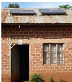
There are two solar panels on the roof of John’s house. The maintenance of the panels is important; they must be kept clean and clear of shadow. If the circuit is broken at any point then the whole panel will not work. Sometimes loose connections need to be fixed. We have trained John to maintain the panel and to do some minor repairs. A cable leads to two charging
